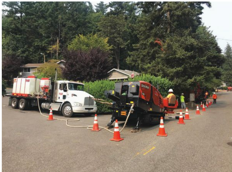
Workers in Bothell, Washington, installing communication conduits.
