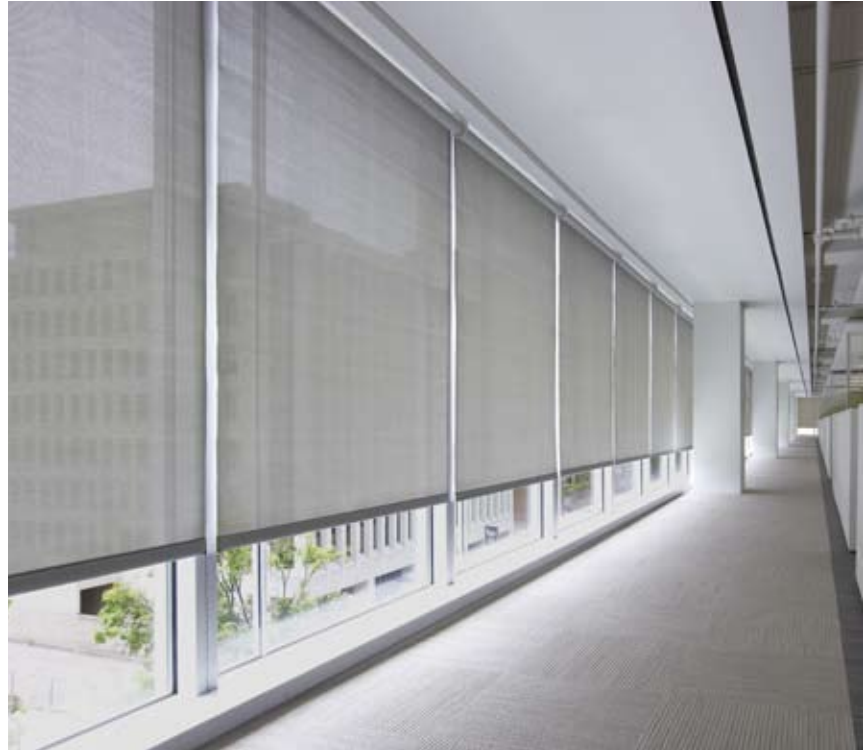
As seen here at the U.S. Green Building Council headquarters in Washington, D.C., in uniform mode, the shades can only be moved to one of five factory-preset or user-defined positions.
