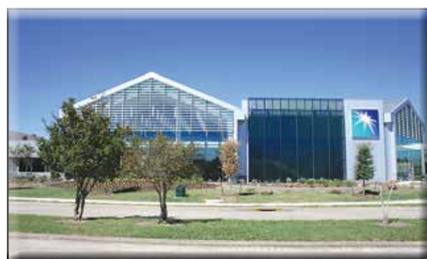
Houston Research Center, Bartlett Cocke General Contractors
