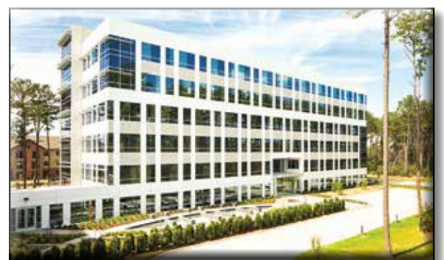
Sierra Pines Phase II, EE Reed Construction LP
