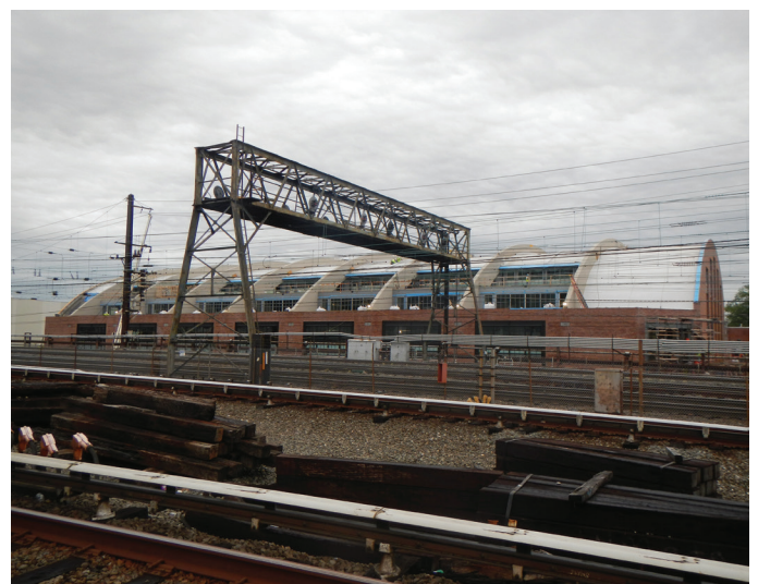
Fig. 3—Sections of the arched concrete shell panels removed to create openings in the roof.
