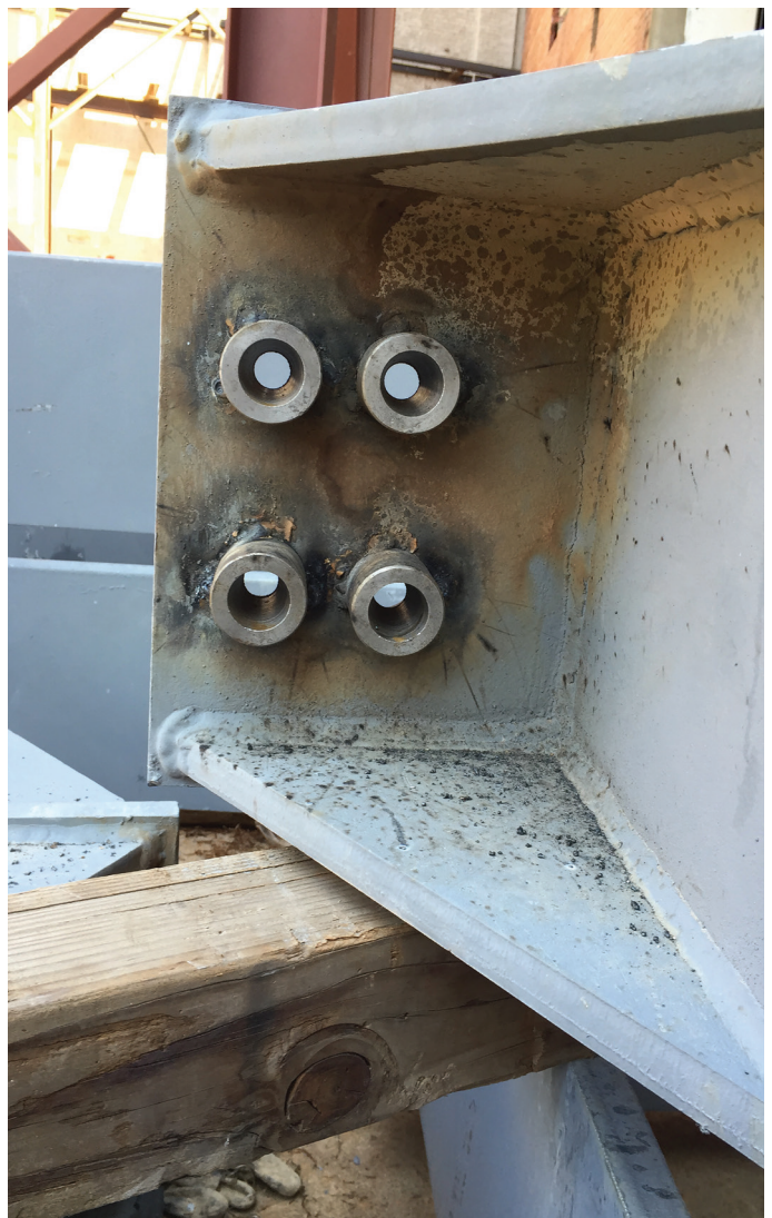
Fig. 6—End block for Barrel Anchors.
