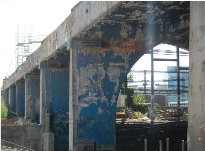
Fig. 5—Cables fixed to anchor blocks located at columns.
