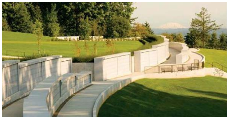
Work performed by Glen/Mar Construction in the $10.6-million expansion of Willamette National Cemetery involved building three columbarium walls. The walls, clad in granite stone, have nearly 10,000 niches designed to hold cremation urns.
