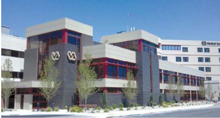
Glen/Mar's work with the VA Sierra Nevada Healthcare System included construction of a mental health outpatient clinic. The $5-million, 15,000-square-foot, two-story medical office building features a glass curtain wall and an architectural metal panel system for the exterior finish, a fully adhered single-ply roof, and glass-tower open areas.
