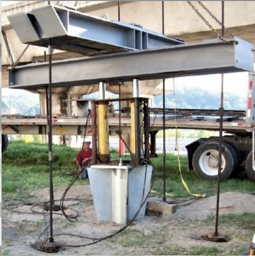
Hydraulic installation of one of our moment foundations for high-mast lighting.
