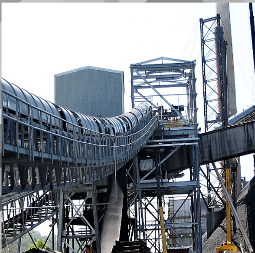
Sammis Power Plant conveyor and transfer tower supported by our foundations.
