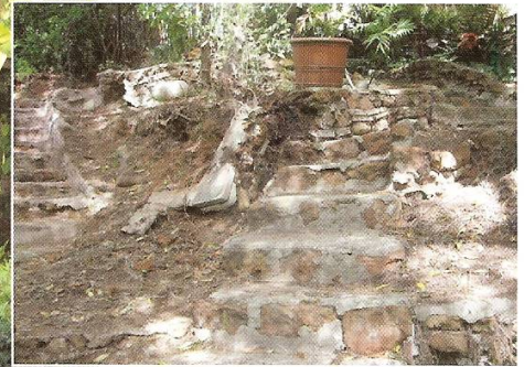
Curvilinear paths and steps of local stone flow comfortably down into the canyon.
