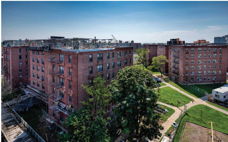
Barami Construction Group responded to Hurricane Sandy in 2012, assisting hundreds of families at the Nordeck Co-Op Apartments in Arverne, New York, by renovating 360 apartments in six buildings.
