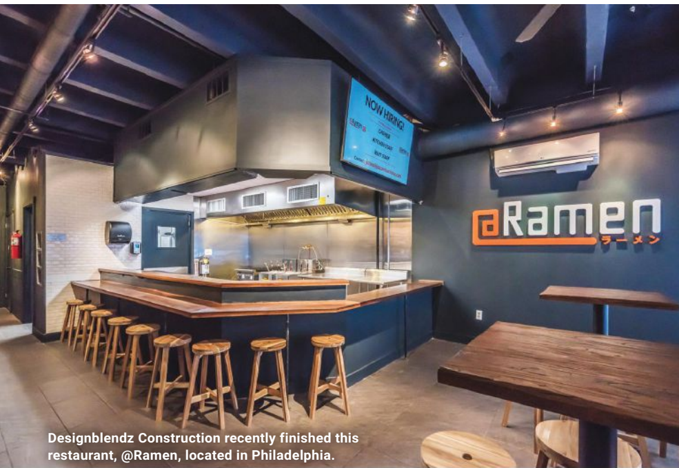
Designblendz Construction leveled and completed rough framing with mechanical rough-ins for a soon-to-be-completed sushi restaurant in Philadelphia.
