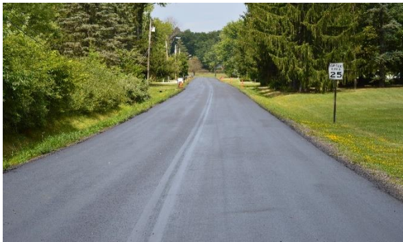
Rejuvenator covered all aggregate and pavement striping.
