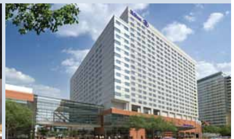
Photos courtesy Brisk Waterproofing
