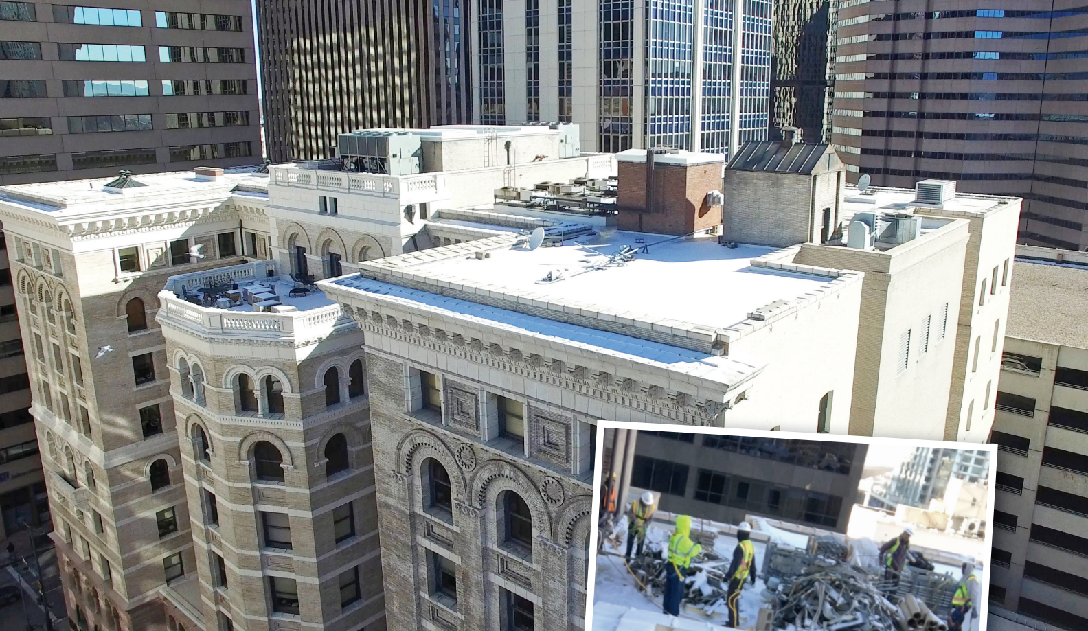
(Top) Lallier Construction, Inc. installed a fully adhered 90-millimeter firestone EPDM rubber roofing membrane on the nine-story Equitable Building located in downtown Denver. (Right) Crew members on the snowy rooftop of the historic Equitable Building in downtown Denver.
