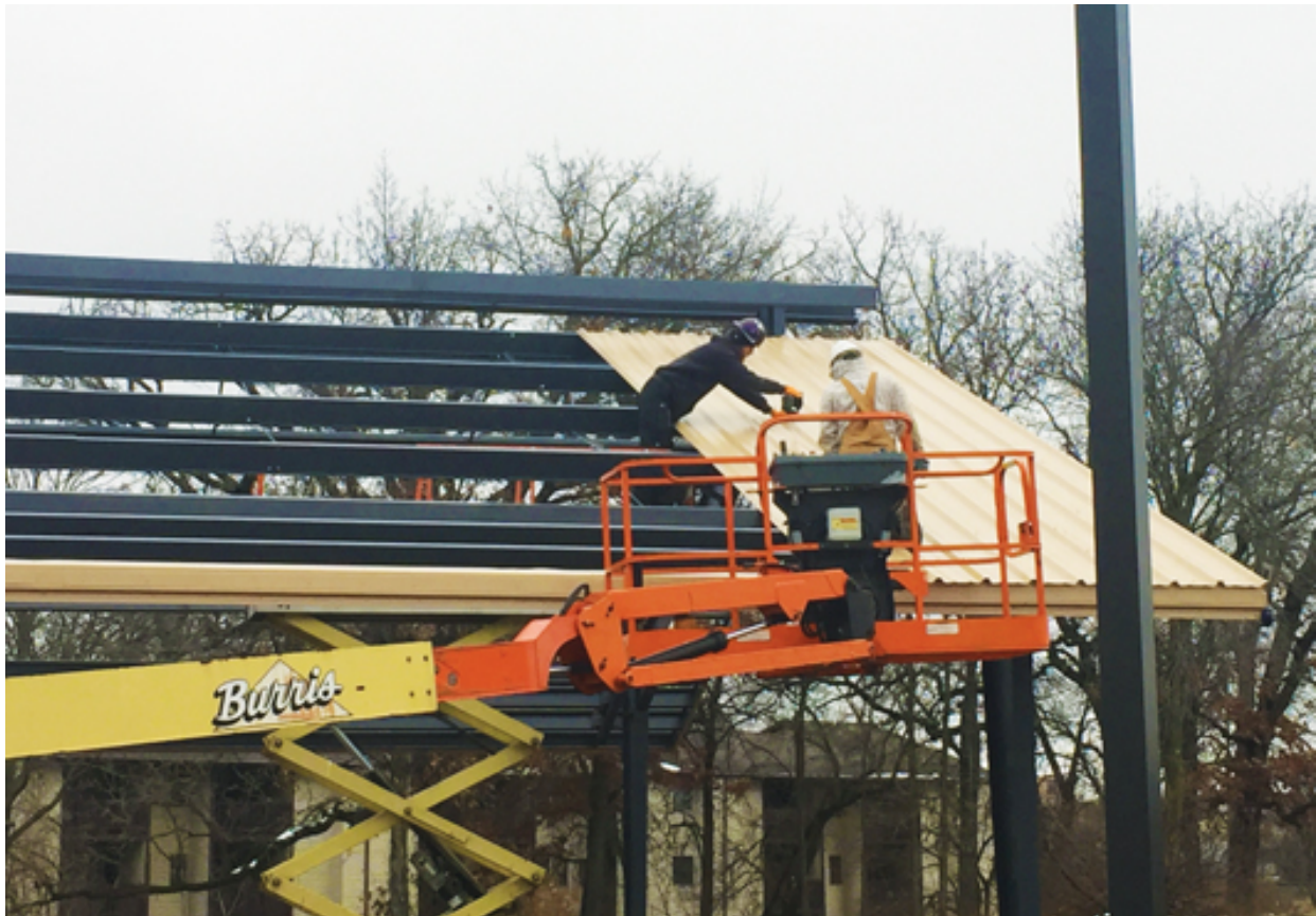
Tim Johannsen, left, and Orlando Diaz, employees of Lake Shore Construction Inc., work on adding the roof panels to the pavilion.
