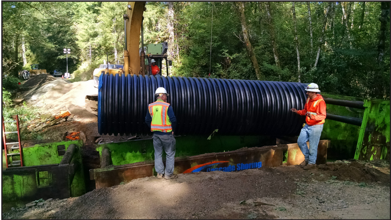
A new 60-inch culvert is gently lowered into place.
