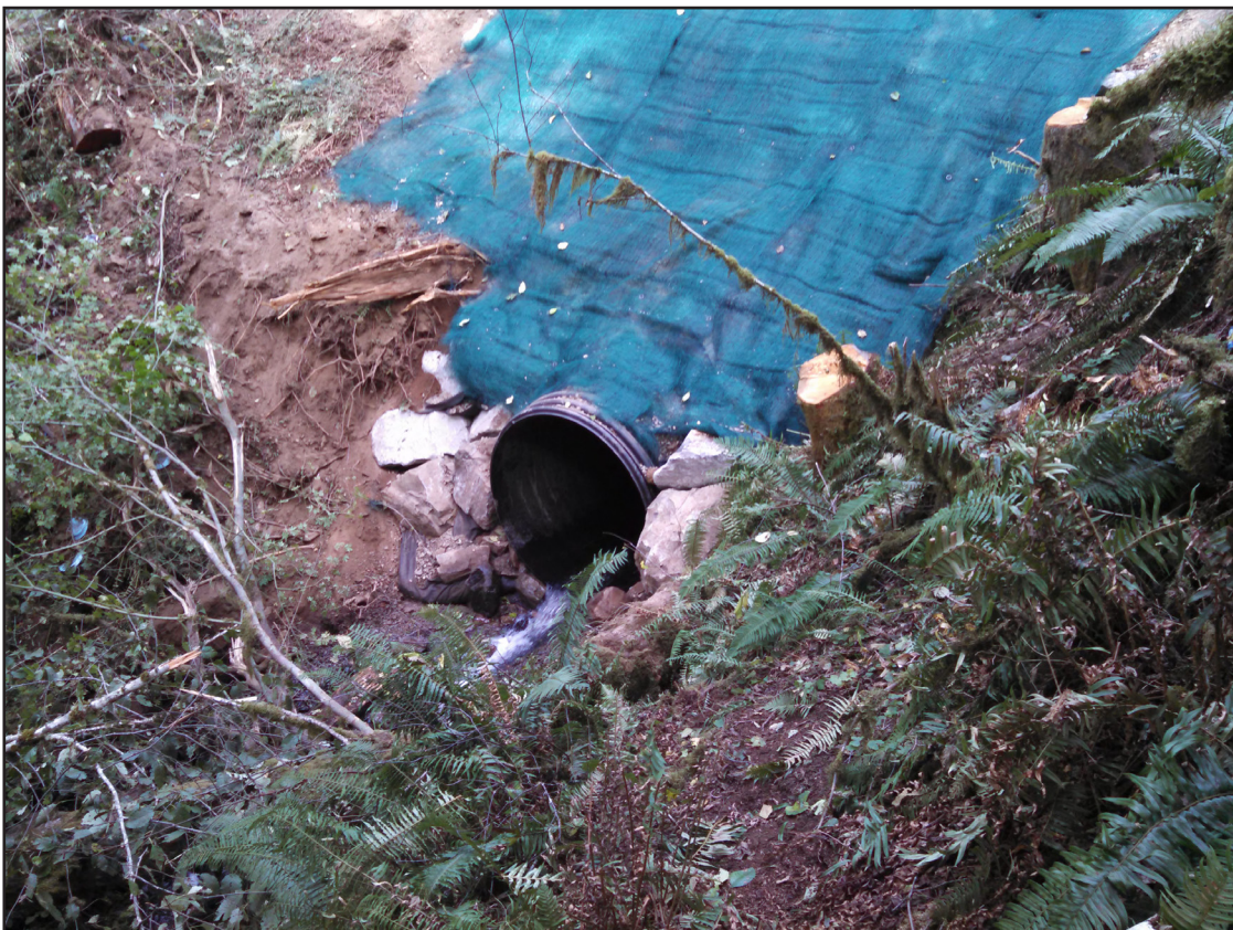
A look at water flowing out of the new culvert.
