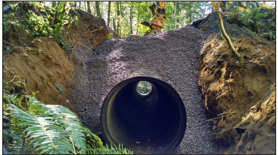
The replacement culvert, shortly after it was put into place.
