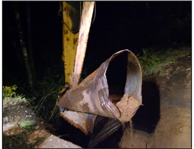
The old culvert that was removed after sunset Friday.
