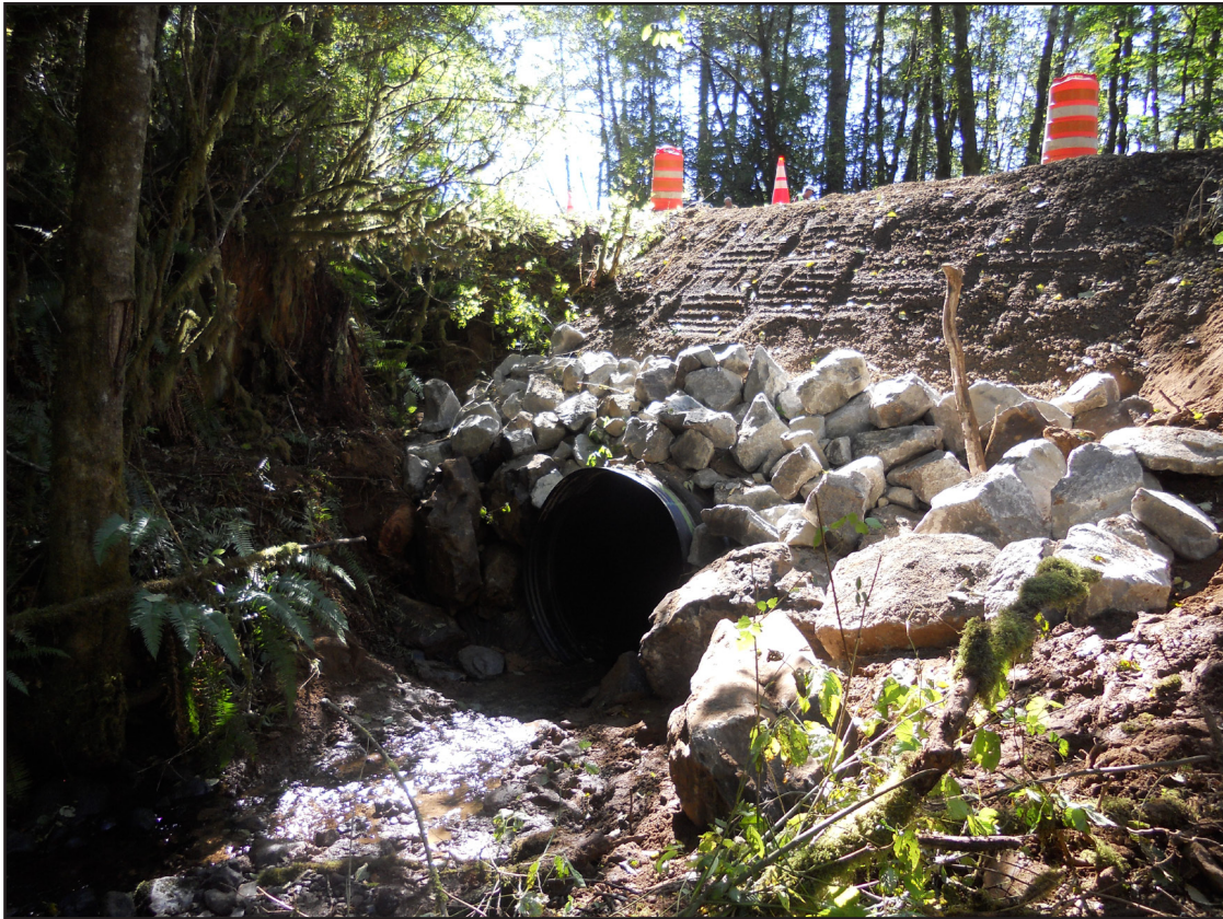
Water runs into the replaced culvert on the upstream side.
