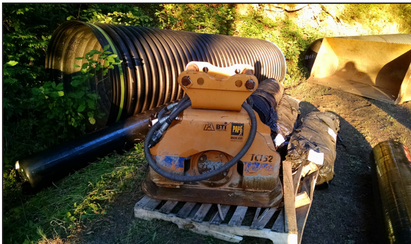
The contractor mobilized equipment even before the road was closed.
