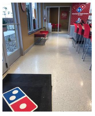
This required abrading the floor with a concrete floor grinder to obtain a proper surface profile. concrete floor also had moisture vapor issues and a fast curing moisture mitigation primer was used as a base coat to prevent moisture from seeping up through the surface and lifting off the epoxy coating. The epoxy coating was self-leveling useful which is concrete floor slabs that may have dips and uneven surfaces. The Domino's
