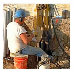
Prior to excavating next to the existing facility, C. T. Taylor's engineers designed and installed a unique shoring system utilizing hydraulic jacking to support the existing building.
