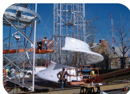
trips between the bracket fabricator and the panel fabricator we were able to reverse engineer the hole locations on the five axis CNC router to mate the two sets of components.
