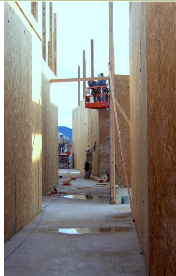
(Above) Sound absorbent SIPs and off-parallel walls create a quieter learning environment. (Left) Nearly completed SIP installation.
