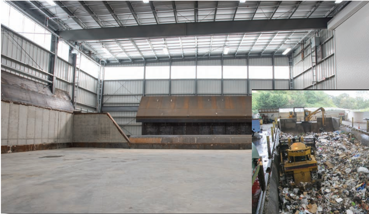
Above: Lift and load pit at the City of Cape Girardeau Transfer Station. Photo courtesy of Cambridge Companies.
