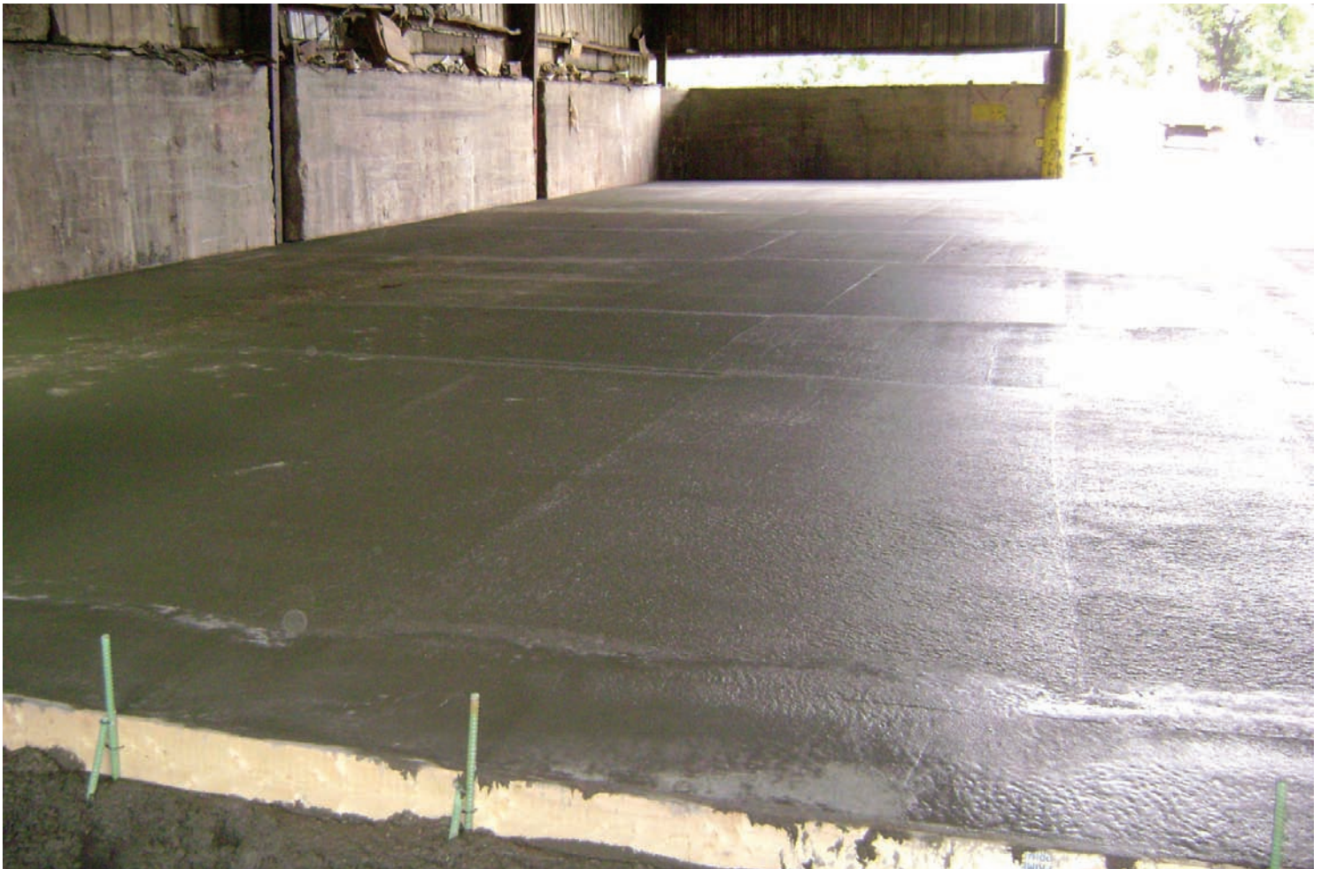
Figure 1: Tipping floor after replacement. Photos courtesy of Cambridge Companies.
