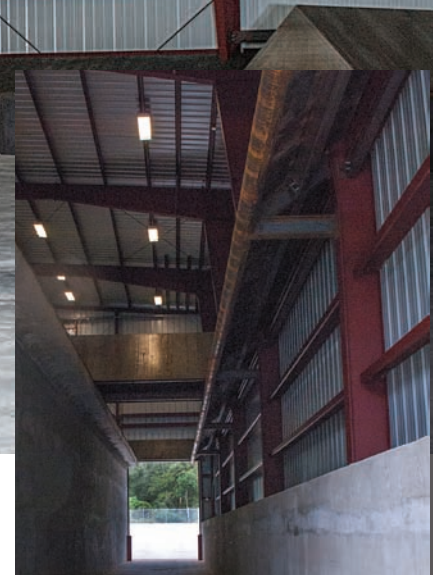
Figure 5 Drive through pit for trucks to transport MSW to landfill.
