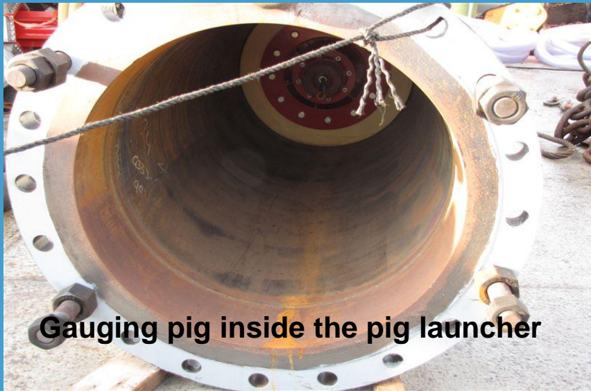
Assembling the pig launcher
