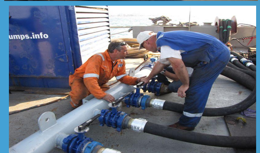
Applying the manifold
