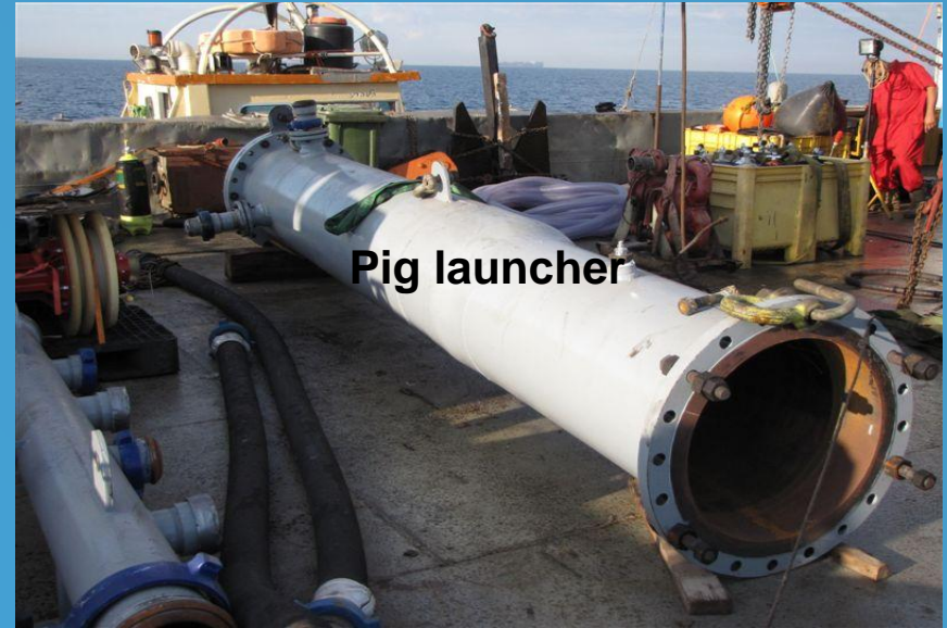
Assembling the pig launcher
