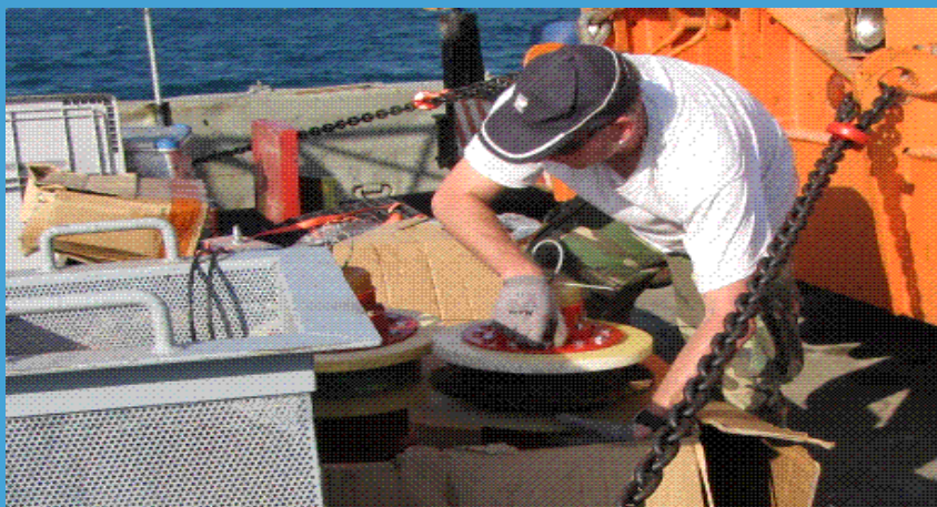
Preparation of the pig launching.
