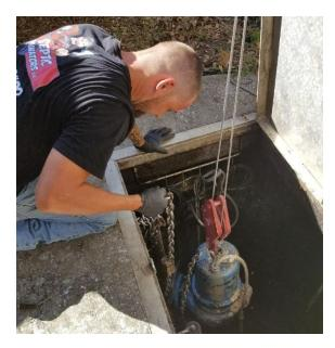
Lift station is another major part of your septic system that you might not be aware of until it stops working. The role of a pump station is to sense and pump waste water from a low elevation to a higher elevation when the natural flow is restricted.
