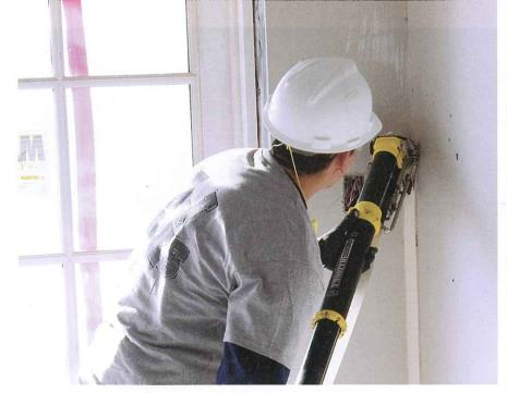
There are more than 20 wear-parts in the typical automatic taping tool set that require replacement in the normal course of operation. For the tool renter, these parts are typically replaced at the time of service, but are often included with the tool in case the contractor keeps the tool for an extended period and needs to swap in a replacement.
