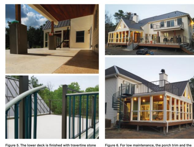
Figure 5. The lower deck is finished with travertine stone that was glued around the perimeter to the steel framing with two-part epoxy. In the field, the pavers were drylaid, and the joints filled with polymeric sand (top). A subcontractor installed waterproof fiberglass walking surfaces on the two upper decks (above).
