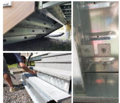
Figure 4. The author modified the original Paverdeck stair framing design, beefing it up with boxed galvanized LGS stringers and joists (top left), and forming the treads and risers with Paverdeck pans (above left). The through-bolts that attached the posts through the stone treads to the Paverdeck pans were backed with large washers (above right).
