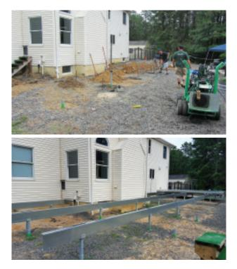
Figure 1. Instead of massive concrete footings, helical piers—each capable of supporting 5,000 to 8,000 pounds—were installed to support the freestanding deck (top). The 6<sup>1</sup>/<sub>4</sub>-inch Paverdeck panels are screwed to galvanized 10-inch LGS steel beams bolted to the brackets on top of the piers (above).
