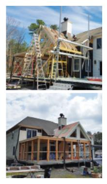
FIgure 3. Support columns for the sunroom bear either on the house foundation or directly on piers (top). The structure was timber-framed with a combination of pressure-treated sawn and engineered lumber (above).
