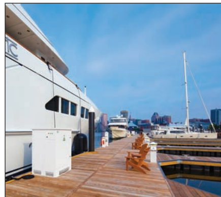
The two phase project replaced all the docks and equipment, while the marina remained open for business.
