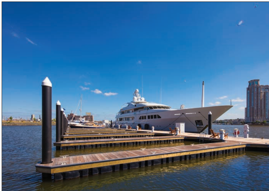
The new marina has 184 slips, from 30 to 100 feet, with side-tie dockage for superyachts.
