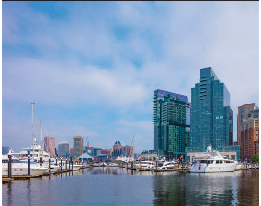
Harbor East Marina in Baltimore, Maryland, completed major renovations earlier this year.
