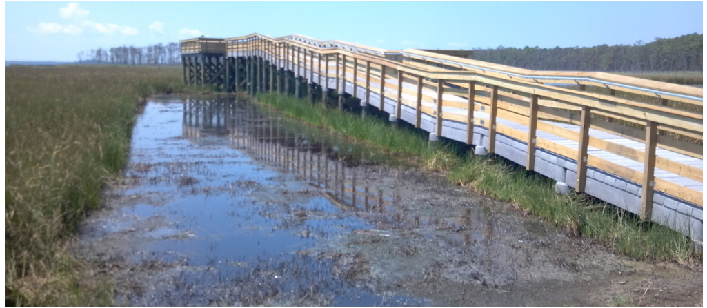
The 210' boardwalk is founded on timber piles.
