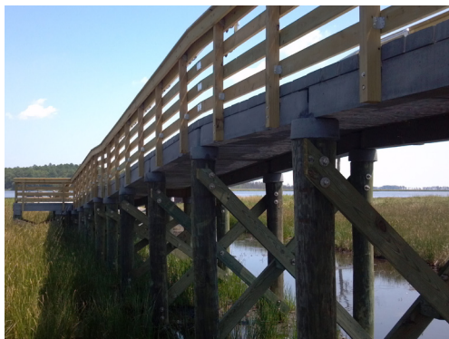
PermaTrak pile caps and stringers (beams)
