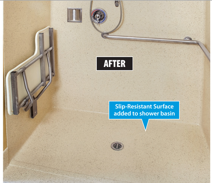
▲ The hotel showers were refinished to like-new condition including the application of Miracle Method's durable Slip-Resistant Surface (SRS).
