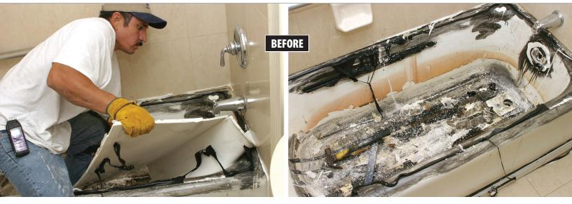
🔺 Miracle Method was able to remove the failed liners, drain the trapped water, remove the mess, and restore 500 tubs to like new.
