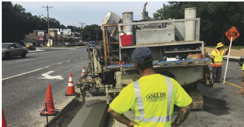
Workers from Anglin Construction Co. oversee the placement of concrete for the median curb along a stretch of Kirkwood Highway in Newark, Del.
