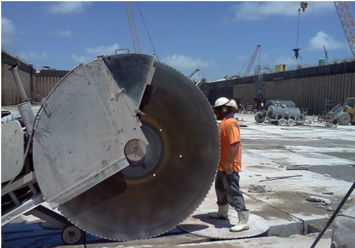
Slab sawing in Texas with a 92-inch-diameter blade.
