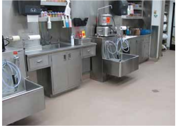
ABOVE ▲ The Raider crew roller-applied the formaldehyde-resistant Wearcoat 100 top coat at a DFT of 4 mils (0.102mm) per coat. "And we put on two coats. We aren't taking any chances," says Tabrizi.
