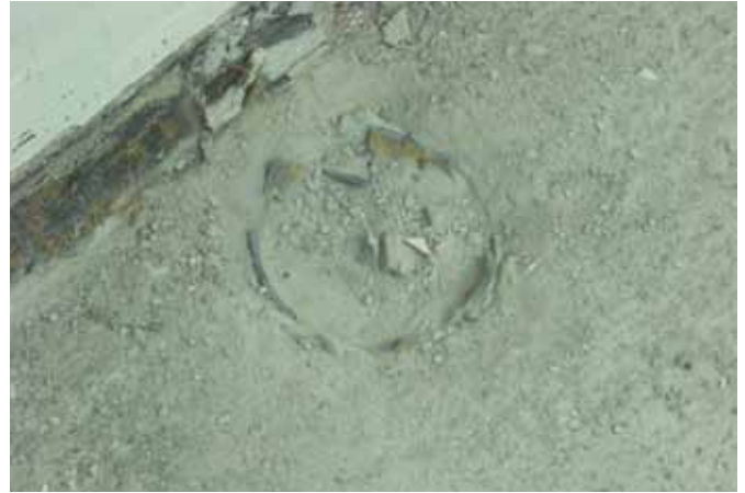
ABOVE ▲ “As we exposed the slab we uncovered an old set of unused pipes that given — the age, setting, and possible use — had to be removed by the mortuary,” explains Tabrizi.
