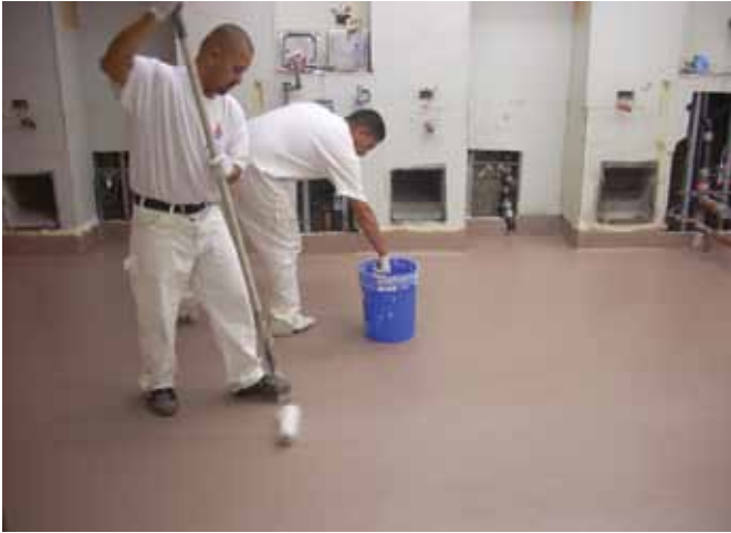
ABOVE ▲ The crew roller-applied 20 mil (0.51 mm) DFT coat of Pacific Polymers' Elastomeric 6001, on top of the 3 to 4 mil (0.076mm-0.102mm) DFT primer and the Mapei system. But they had only just started.
