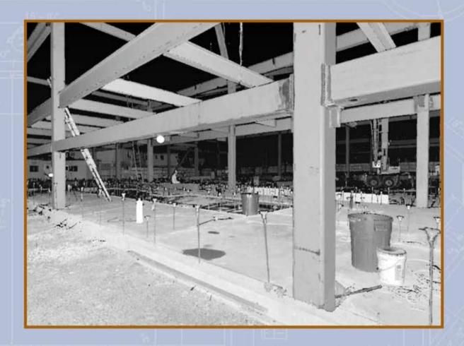
Corinthian Data Capture laser scans the entire site using phase shift laser scan metrology. We capture trillions of points of data. Although we were contracted to document the anchor bolt locations, as you can see we captured:
