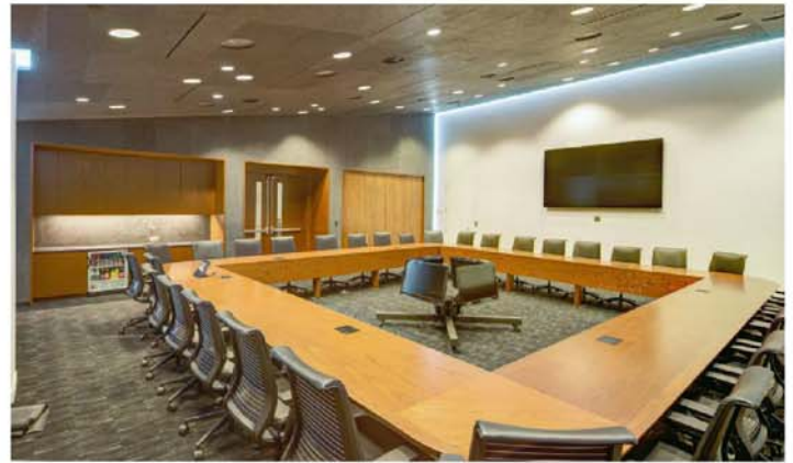
Our scope of work in the Board Room included the 20'x20' conference table, metal 4-screen monitor stand, walnut beverage bar with granite top and back-splash, walnut entry floor, wall paneling and ceiling paneling. The walnut was finished using a medium walnut stain with 60 sheen clear lacquer; we also finished the door jambs and doors.
