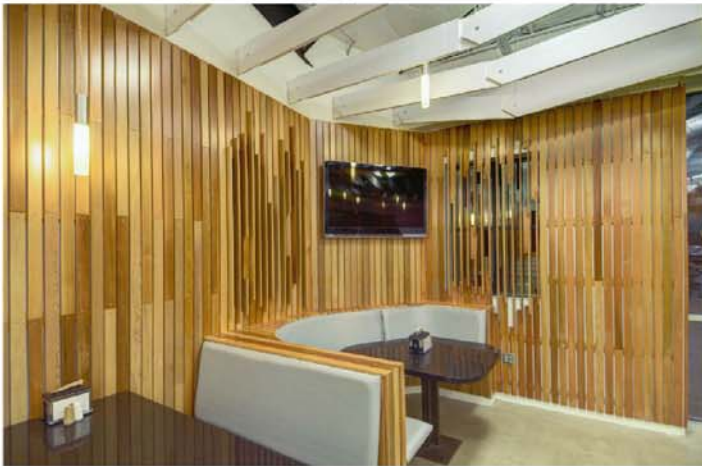
Close-up of the cedar over windows and banquettes. 1x3's flow from wall to top of banquettes to floor. 15,000-linear feet of Western Red Cedar was used, it took 25,000-pan head stainless steel screws to install.
