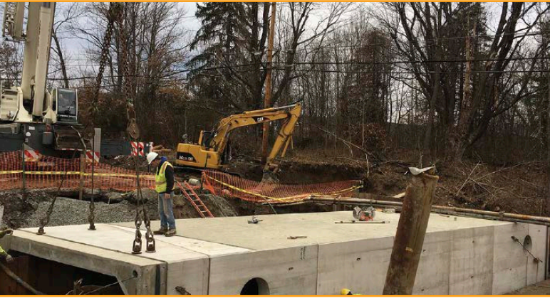
Marshall Hill Rd. Culvert, West Milford
