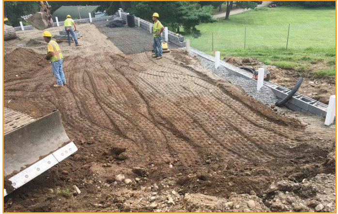
NJ Fireman's Home, Boonton
