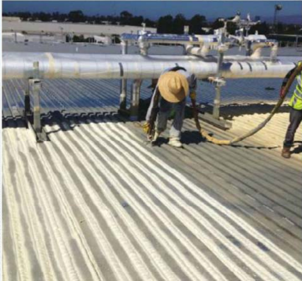
The crew used 115 days to install the new 172,000-square-foot (15,979 m 2 ) roof system onto the Robinson 22-gauge metal "B" deck with flutes. After cleaning the deck, it was onto the coatings system.
