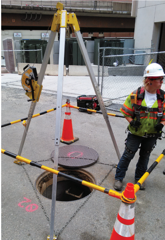
Dangerous confined space entries are made safe with the right personal protective equipment and safety measures.
