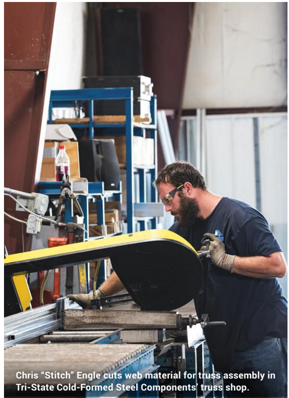
Daryl Dearing assembles metal roof trusses in Tri-State Cold-Formed Steel Components’ truss shop.
