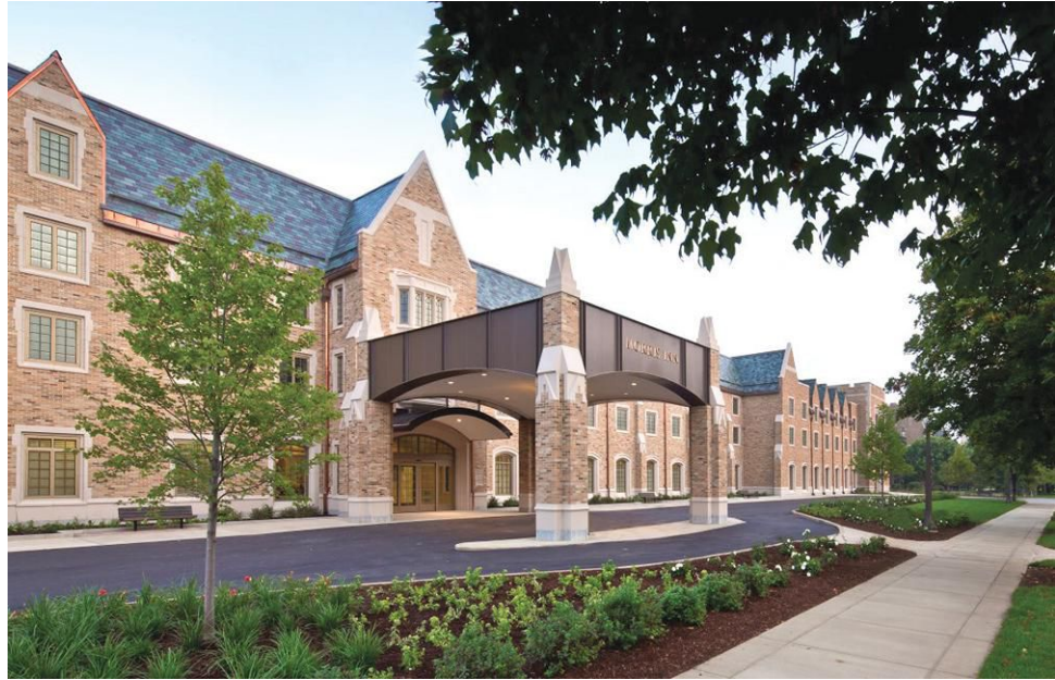
Morris Inn is one of several structures on the Notre Dame campus built with Tri-State’s cold-formed components.
