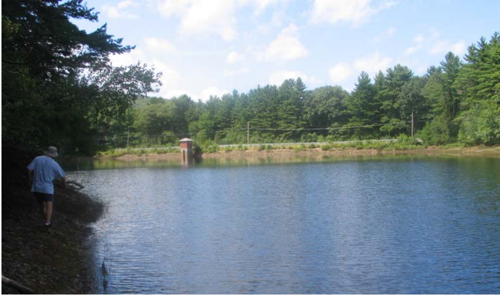
Figure 1: Subject of geophysical investigation viewed from reservoir side.
