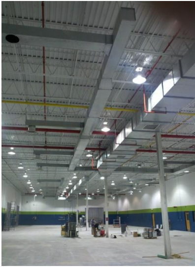
Office & Industrial Painting: walls, ceilings, pipes, floors interior and exterior
