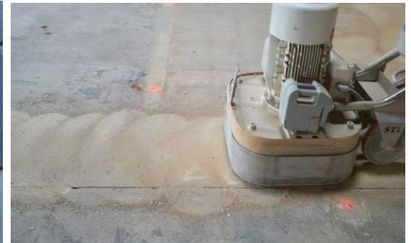
Surface Prep/Concrete Polishing - Adhesive/coatings removal
