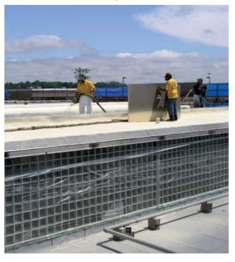
was access to all sections of the roof and the company had to run hose as long as 500 feet from the machine. Since the H-50/60 Gusmer machine is capable of spraying up to 60 pounds per minute, heating large amounts of material so that it's still around 120 degrees F when it emerges 500 feet away was a challenge. Piccione took the machines to Gusmer, which upgraded the heated hoses and couplings while installing an innovative hybrid heater in the unit.
