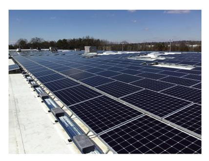
The 925 SunPower solar modules on a Panel Claw support system complete a 302 kW production capacity, which, over the course of a year, will provide power in excess of current consumption—approximately 105%—and will help draw quarterly checks through SREC's purchased on the utility market and monthly credits directly from the electric utility.
