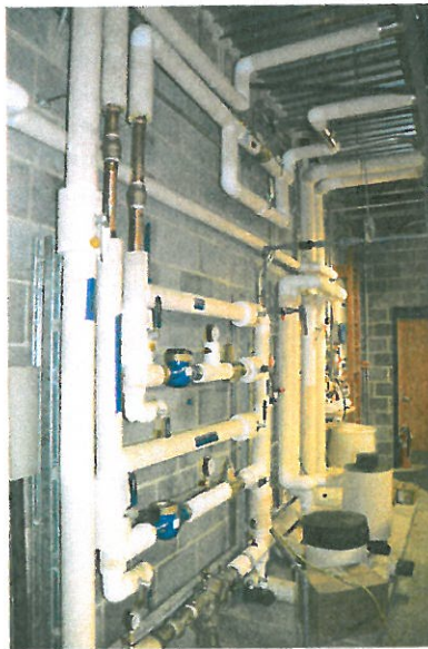
The job included piping rework.
