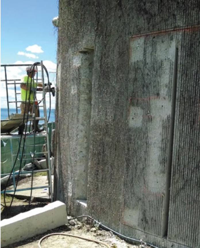
The contractor created six openings 9.5 feet tall in the exterior wall.
