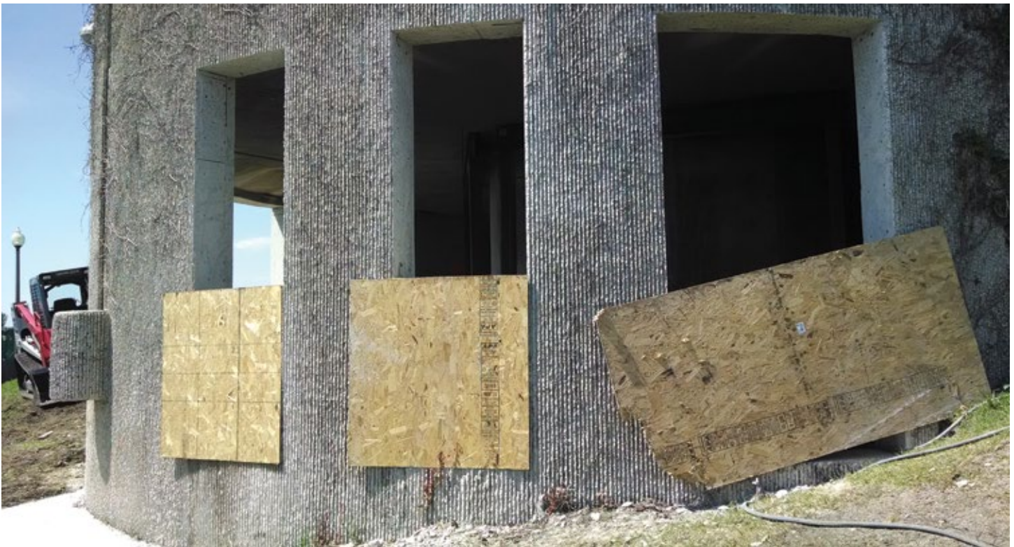
A wall saw was used to cut through the 14-inch-thick concrete.
