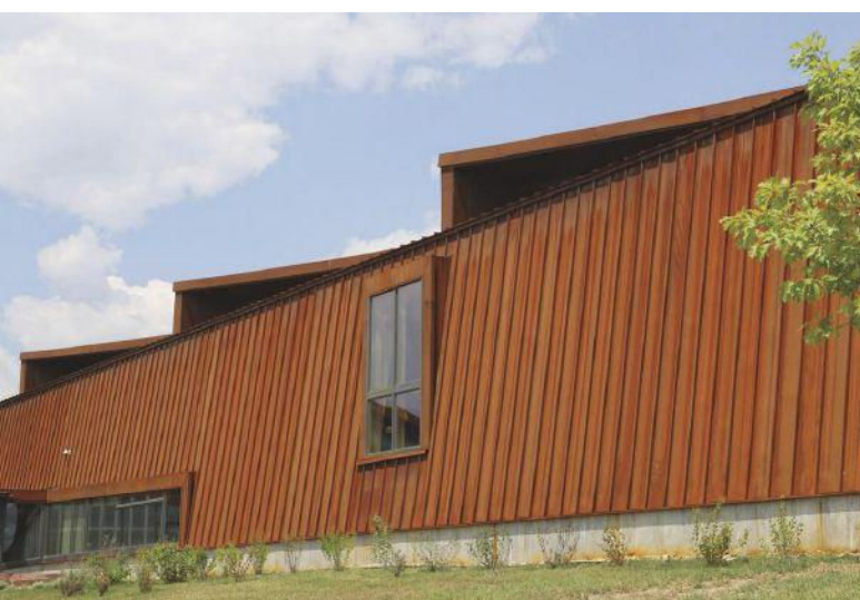
Premium Lock 200 mechanical panels in A606 rusty steel.
