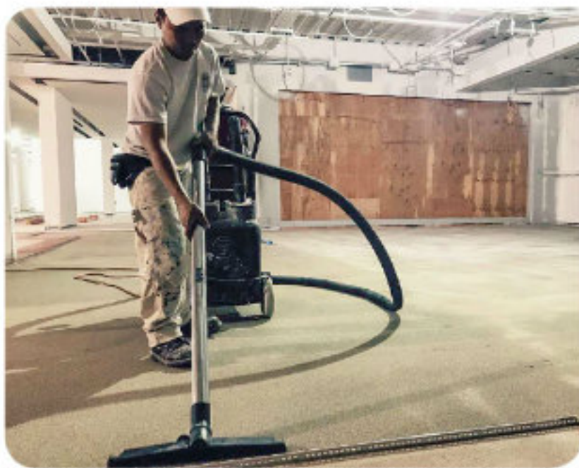
An overlay is a floor finish that's poured and placed on top of an existing substrate. It is important to prep, prime, and clean the floor prior to pouring an overlay.
