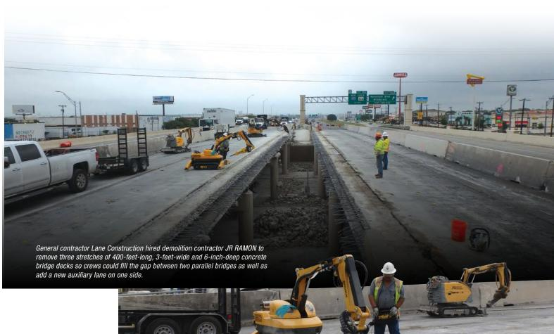
A JR RAMON operator uses the Brokk 120D's remote control to direct the powerful and precise three-part arm with an Atlas Copco SB 152 breaker to remove bridge deck concrete while avoiding the underlying rebar.
