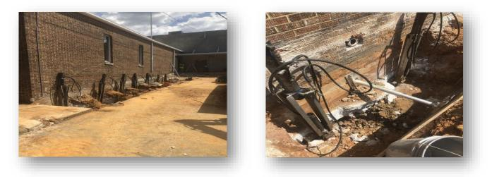
During the lifting process a series of lasers and monitoring devices are being used to watch the lifting process. During lifting there are times that adverse reactions occur to prevent lifting successfully like rotation of the wall which is why we stopped at only 2 inches of lift. Ultimately the foundation is stabile and cosmetic repairs will be made to the structure.
