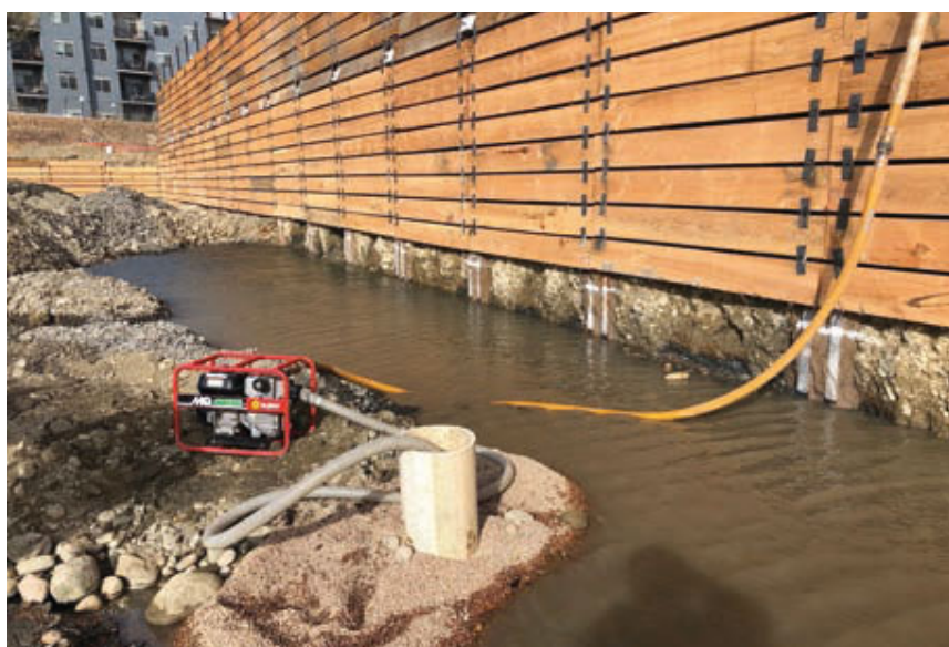
What a difference a day makes. Dewatering Revé's south excavation using filtered portable sump well installation. Photo by David Giles, TerraFirma Earth Technologies, February 2019.
