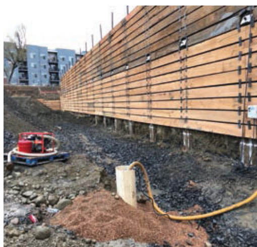
What a difference a day makes. Dewatering Revé's south excavation using filtered portable sump well installation. Photo by David Giles, TerraFirma Earth Technologies, February 2019.
