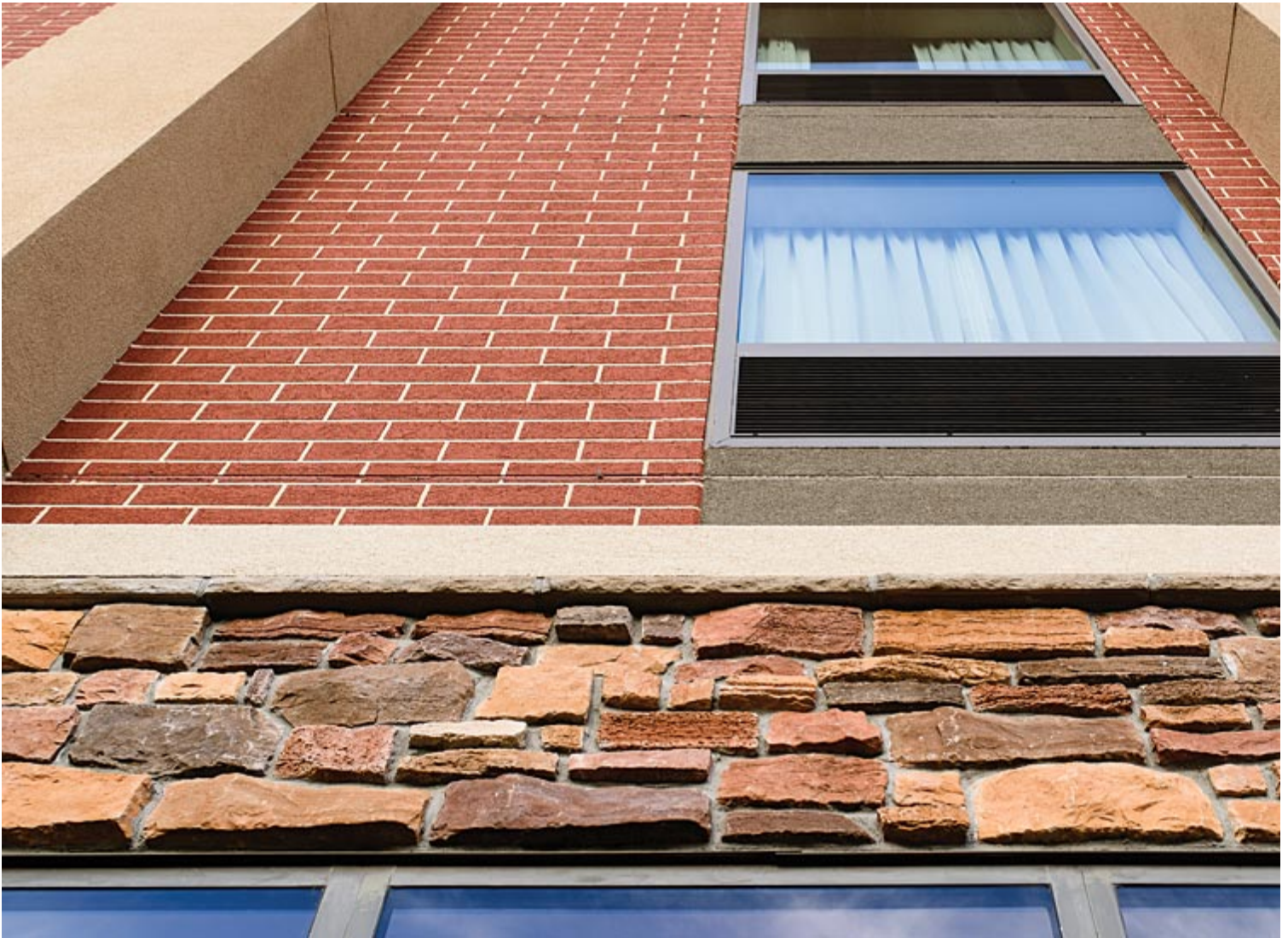
A close up of post renovation exterior with new windows and mix of cladding materials.
