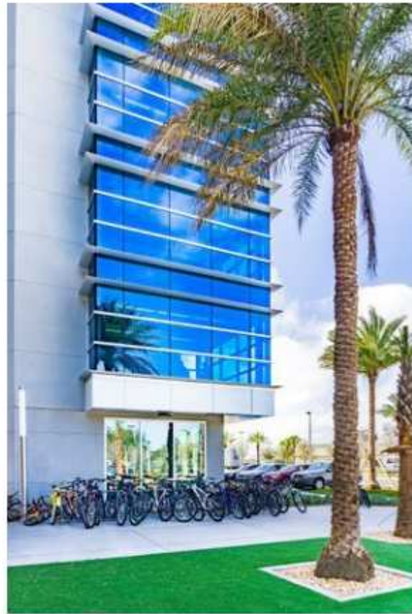
Tubelite's systems feature Viracon glass to help manage Florida's sunshine, maximizing the window-to-wall ratio and exceeding current domestic energy code requirements. Photo: Charles LeRette
