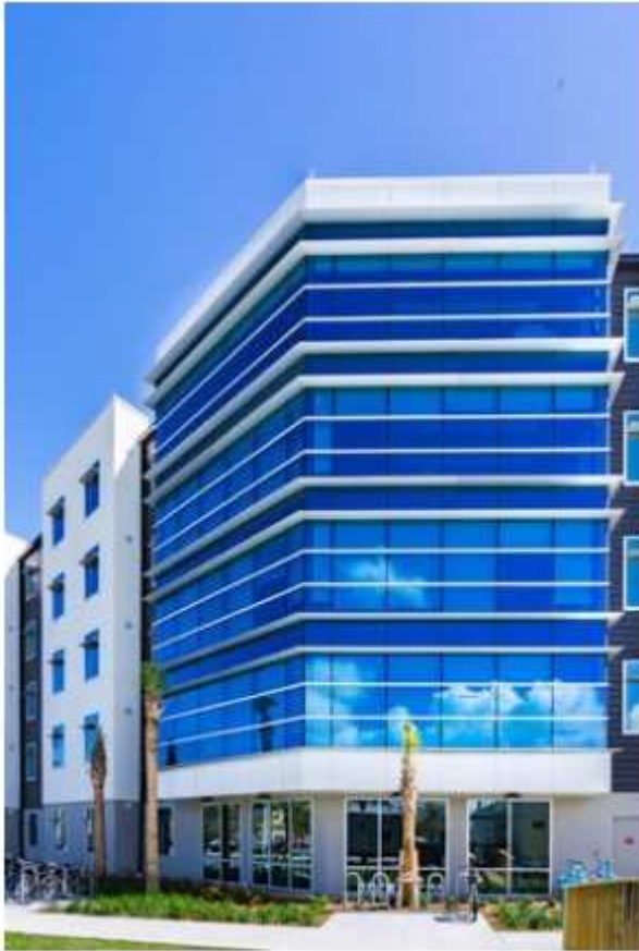
Tubelite provided Tab with its 400CW and 400SS Series curtainwall systems, 4500 Series storefront systems, and Medium Stile Door leaves. Photo: Charles LeRette Photography
