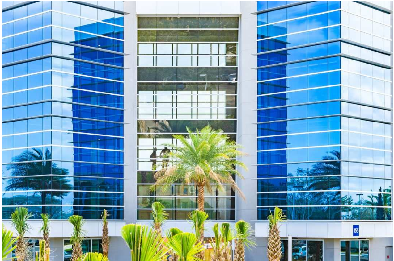
Embry-Riddle Aeronautical University, Daytona Beach campus, New Student Residence Hall. Tubelite Inc. provided window, curtainwall, storefront and entrance systems, and an airfoil fin. Photo: Charles LeRette Photography
